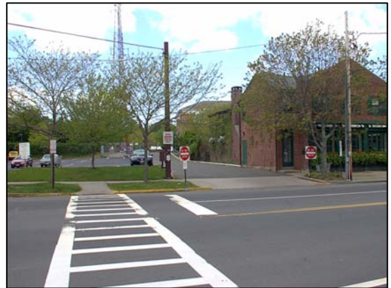
Existing crosswalk on North Main Street East Hampton, New York
