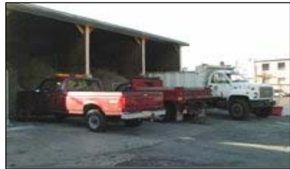
Existing Fort Lee DPW Yard New Jersey
