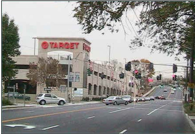
View of Sanford Boulevard shopping center from the east Mount Vernon, New York
