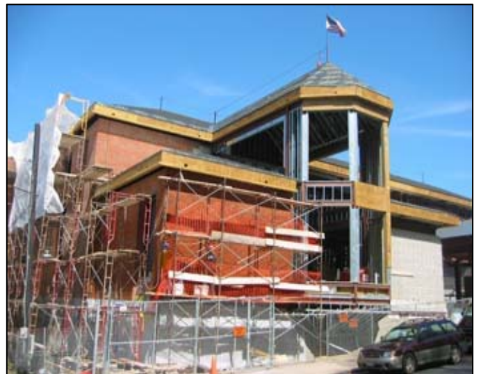
The New Public Library Under Construction Ossining, New York
