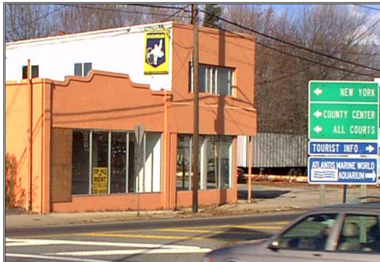
Former Tire Craft store at traffic circle in Riverside
